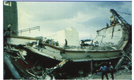
El Salvador Earthquake, Destroyed
